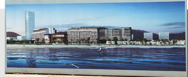
Project Name: INTERCONTINENTAL HOTEL Location: Ha Long Bay Customer: Alliance Co. Completed: On-Going Scope of Work: Gypsum board & Painting work
