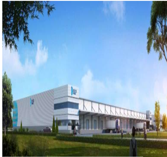
Project Name: SLP FACTORY Location: Nam Dinh IP, Hai Phong, Ha Noi Customer: Ricons Completed: 2022 Scope of Work: Repainting PU
